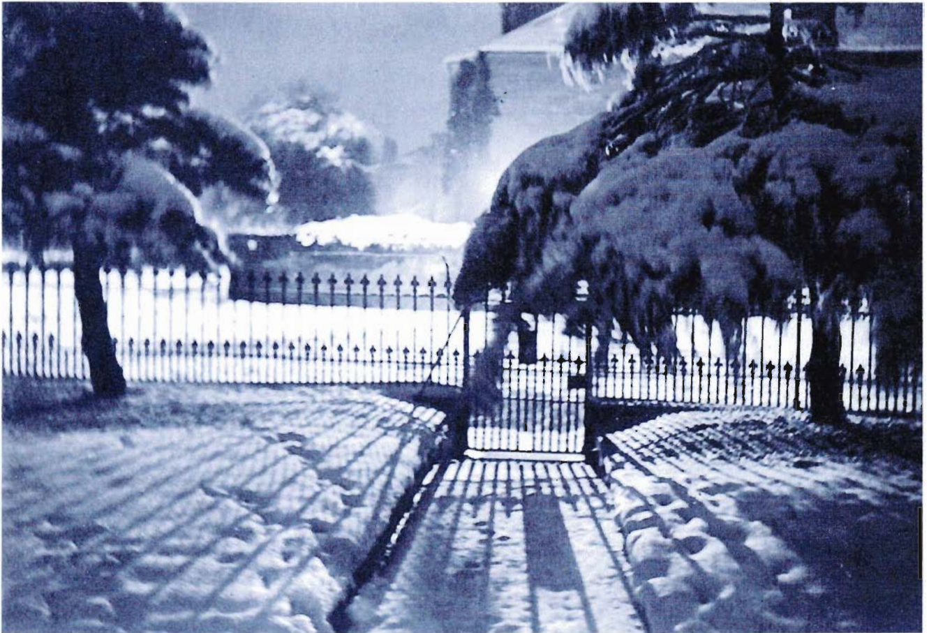
Traditional Railings in Blacket Place
